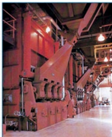
• Solid Fuel LaMont's in a District Heating Plant •
