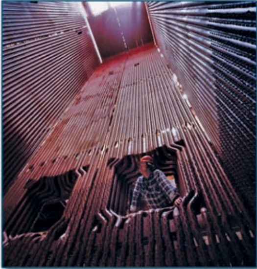
• Membrane wall furnace with two burner openings in an RDF fired boiler •
