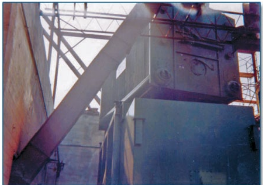
• A - Boiler being lifted into place •
