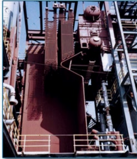
• 2-Drum Boiler being erected showing pendant Superheater •
